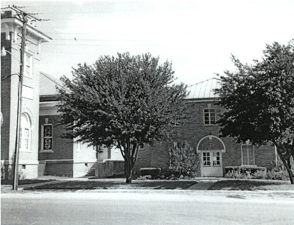
South elevation of addition, with original building on left
