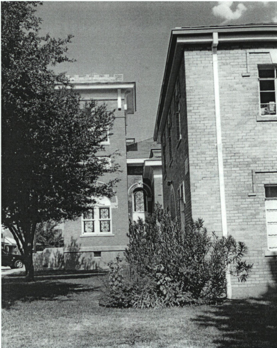
East façade, including SE tower of original structure on left and addition on right
